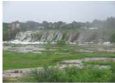
2. Water overflow at the dam wall
